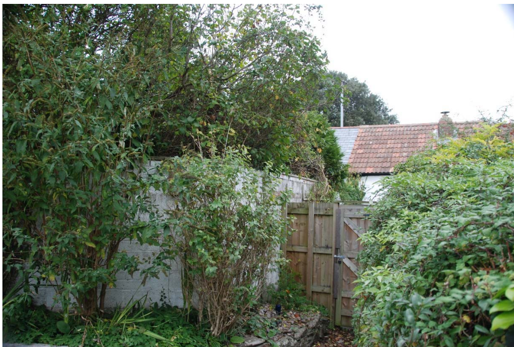
5c : Concrete block boundary wall between 4 & 5 Church Hill.
